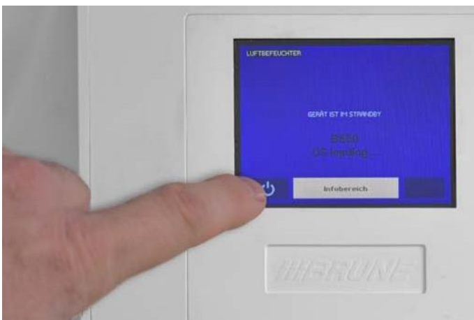
Fig. 5.2.1: Switching on the unit
