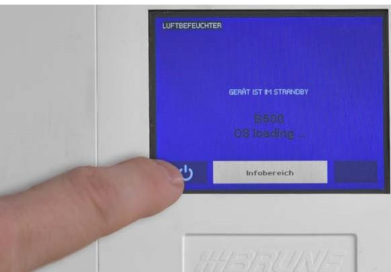
Fig. 4.3.6: Switching on the humidifier
